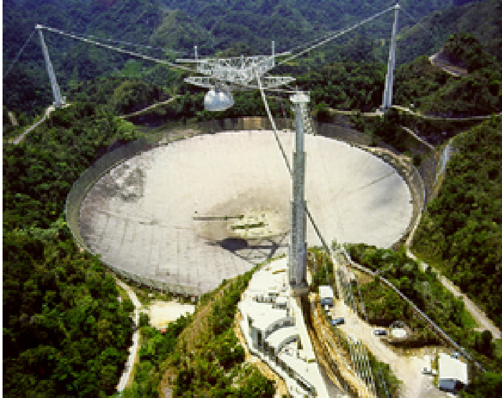
Figure 6: A spherical fixed main reflector antenna at Arecibo, Puerto Rico, USA, 305 m diameter.
