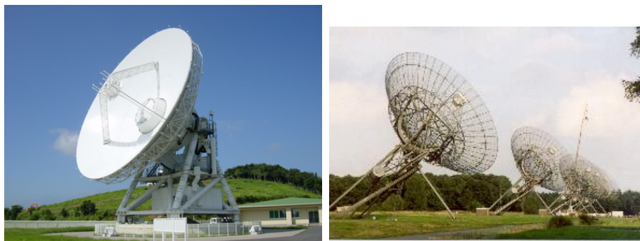
Figure 5: Alt–Azimuth mount antenna at the VERA Iriki station, Japan (left), and Equatorial mount antennas in the WSRT, the Netherlands (right).
