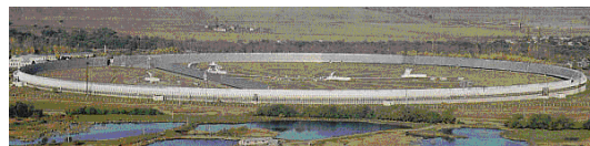
Figure 4: The partial cylindrical paraboloid antenna RATAN-600, Russia.
