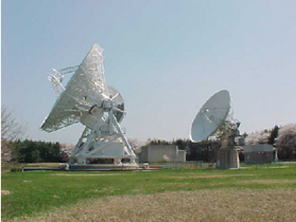
Figure 7: Wheel & Track (left) and Yoke & Tower (right) antennas.
