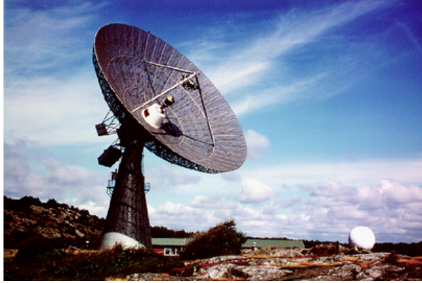
Figure 9: A cm-wave antenna at Onsala, Sweden, 25.6 m diameter.
