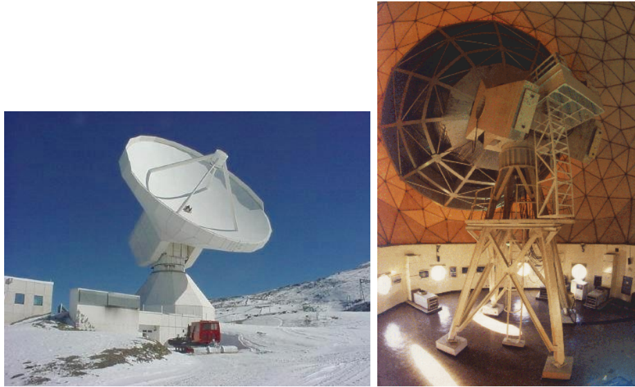
Figure 10: IRAM mm-wave telescope, Spain, 30 m diameter (left), and radome-covered TRAO 14 m mm-wave telescope at Daejeon, Korea (right).
